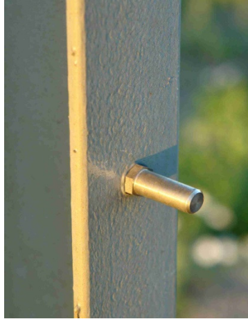
Fig. 1. Track axis reference point and at the same time railway geodetic network point fixed to a traction current pylon
